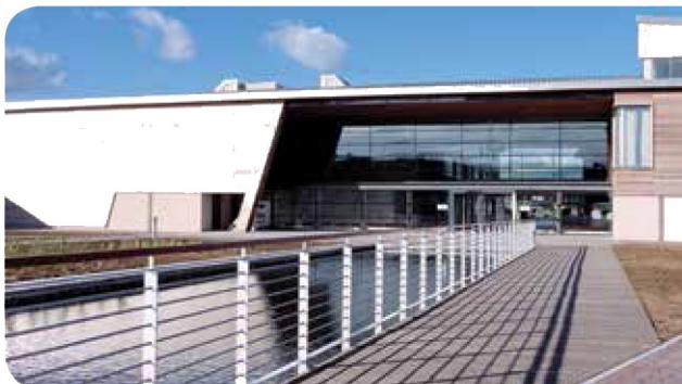
National Maritime College of Ireland (NMCI)
